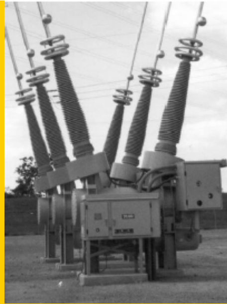
Fig. 13-25 SF_6 circuit breaker [5].
